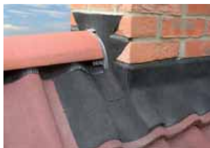
Ubiflex Black - chimney flashing over profile tile
