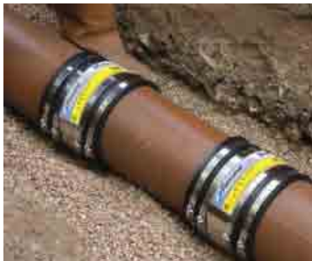
Two Flexseal SC200s, replacing a section of DN150 vitrified clay pipe
