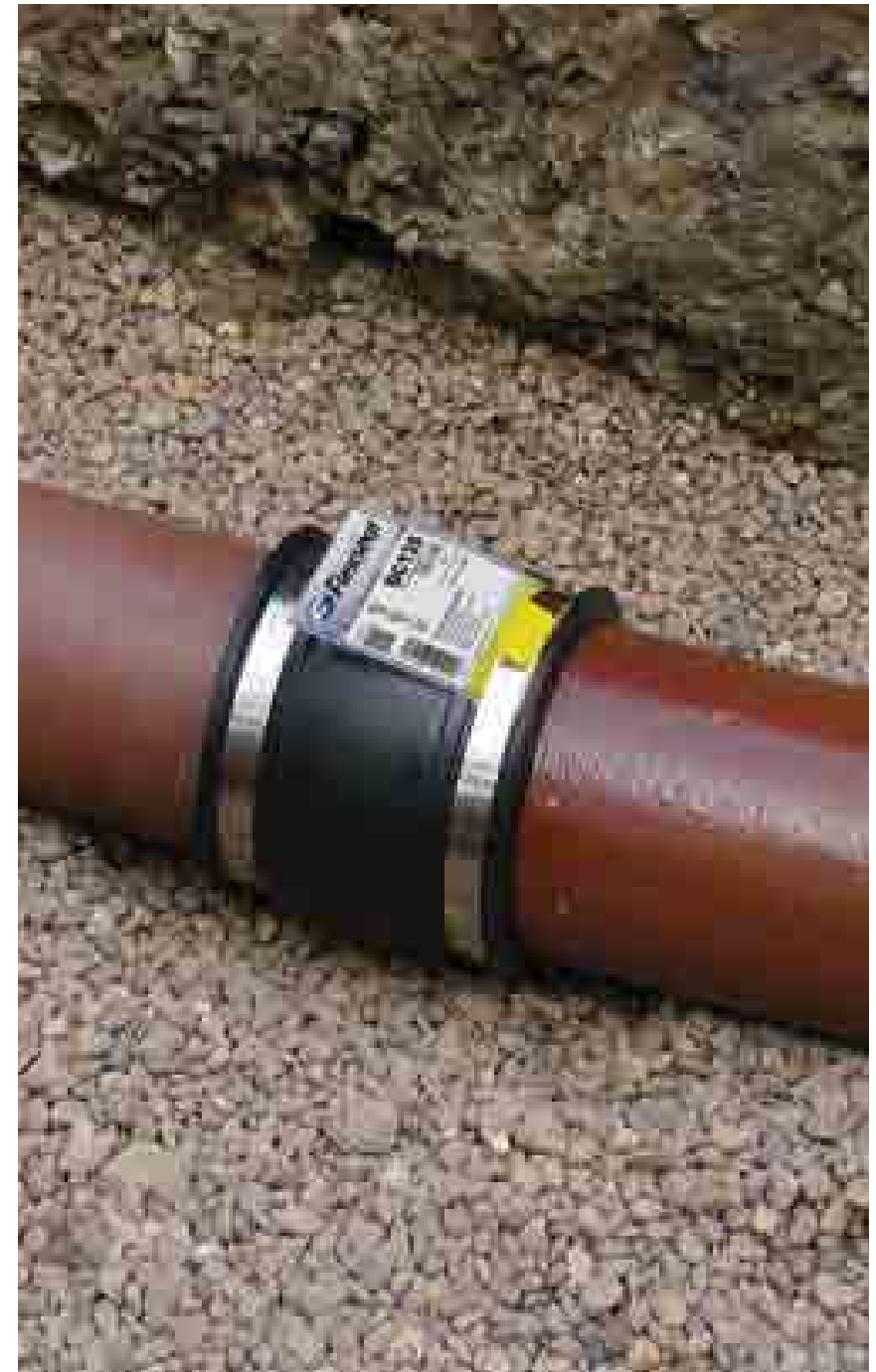
Connection of a DN100 Supersleve to a DN100 salt glazed clay
